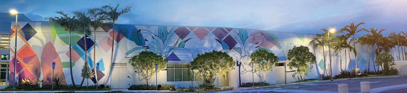
Photo: North County Service Center
